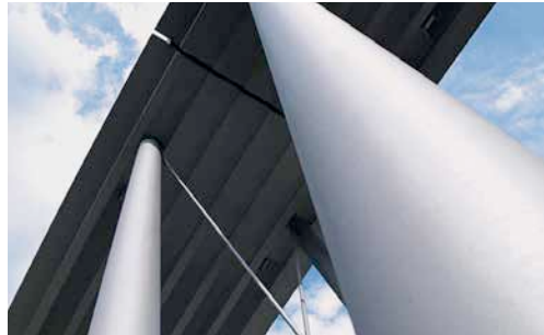
Bridge construction with textile reinforcement
